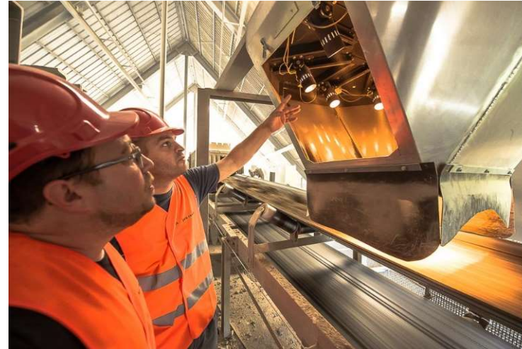
Inside view during operation
